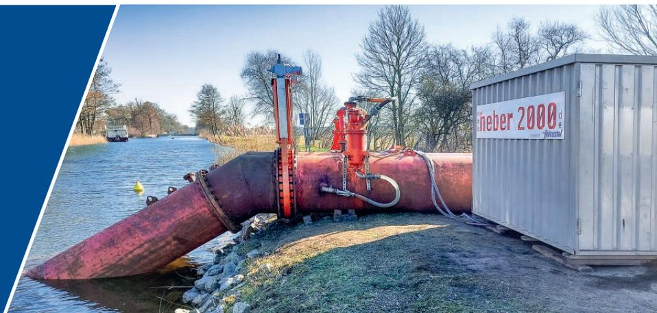
The **heber 2000** uses the natural slope and its water level difference as an energy source and therefore does not require any external drive energy. External energy is only used for commissioning and maintaining operational readiness. Even in the event of a power failure, the system continues to pump for a longer period of time. This principle is therefore a particularly economical and reliable method of transferring large quantities of fluid.
